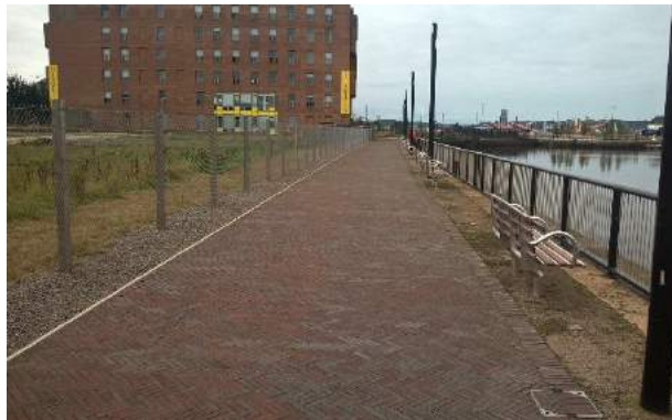
Plate 3.11 Footway / Cycleway on South-eastern side of Roath Dock
