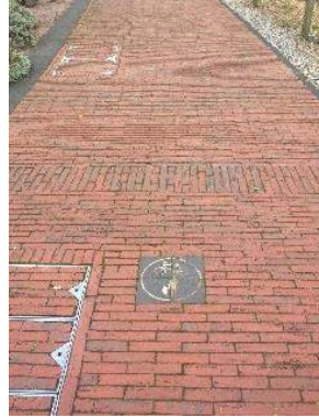
Plate 3.9 - Shared Footway / Cycleway Porth Teigr Way
