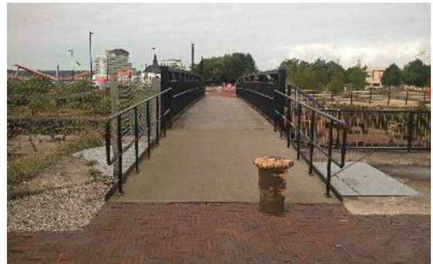
Plate 3.12 Footway / Cycleway on South-western side of Roath Dock
