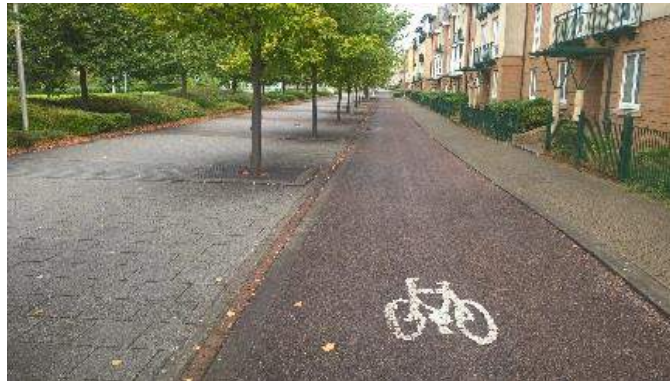
Plate 3.16 - Shared Footway / Cycleway Lloyd George Avenue
