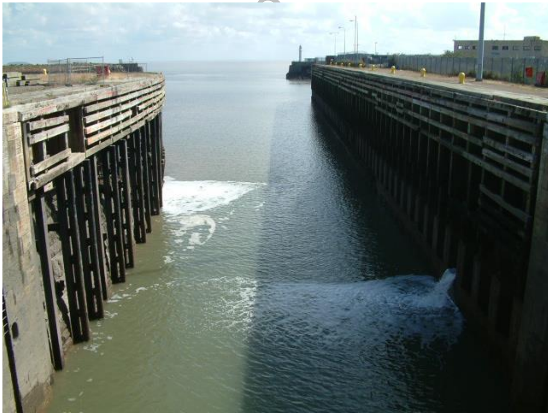
No 3 dock Basin entrance
