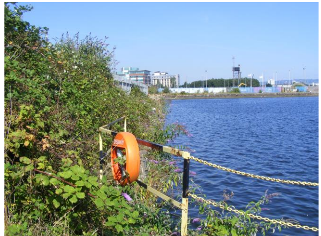
Figure 3 - Looking north-eastwards from the eastern boundary of the Site across the Roath Dock
