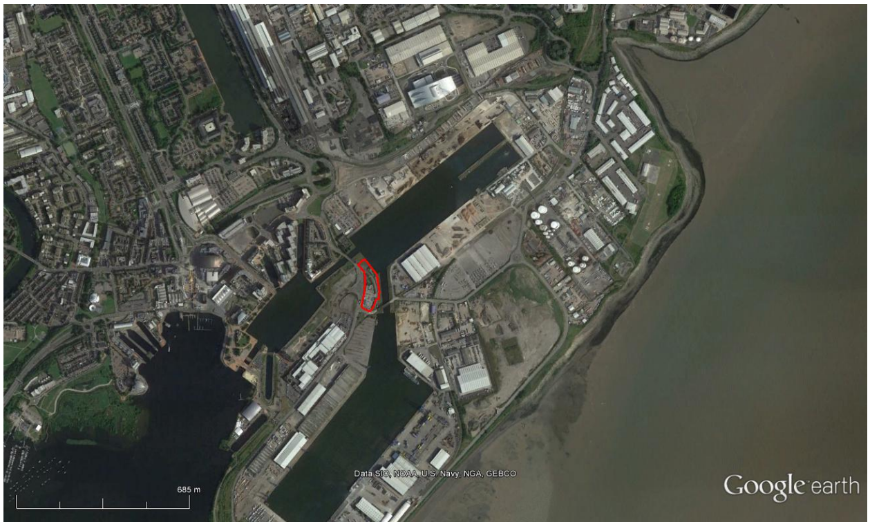
Figure 1 - Aerial image of the site. © Google Earth 2017, imagery dated 16/08/2016
