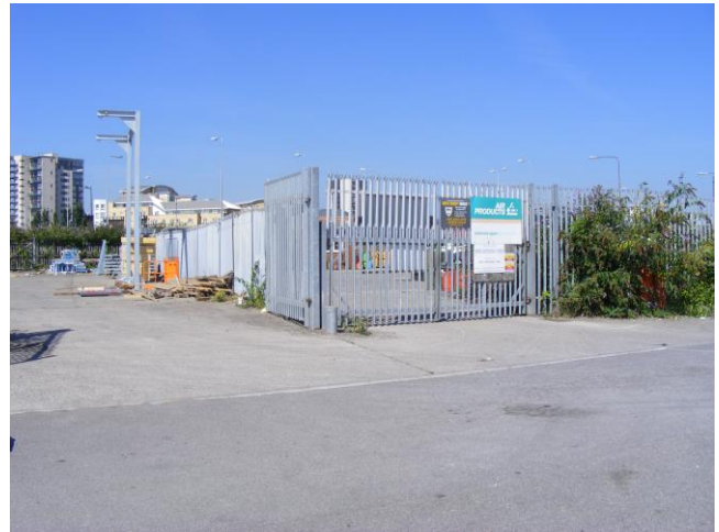
Figure 9 - View towards tenanted compound at the southern end of the Site
