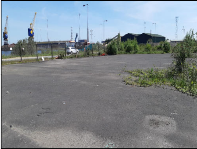
Photograph 1: Looking south west across an area of hardstanding (HS1).
